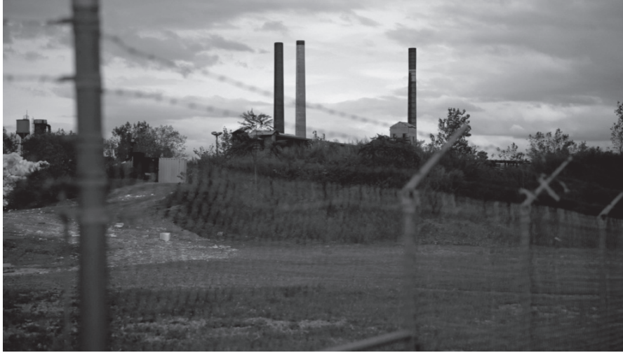
Tonawanda coke plant in New York. Photo Credit: John Poole/NPR
