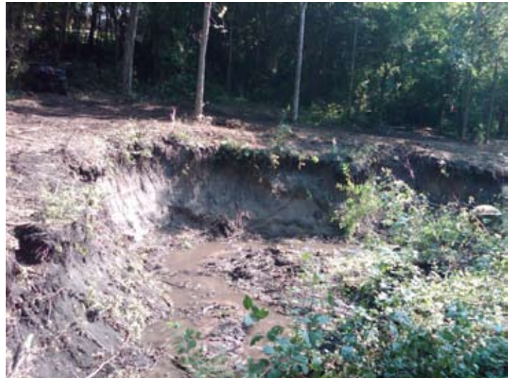
Significant erosion from the Utica Ravine in the City of Savage was a large source of sediment to the turbidity-impaired Credit River.
