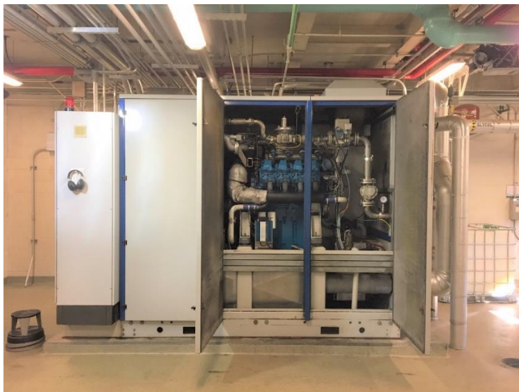
Figure 4. Leibherr combined heat and power engine. Source: DTMA.
