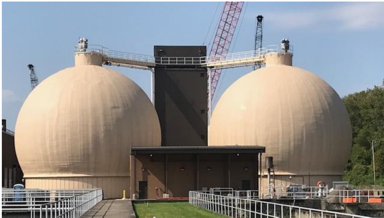
Figure 3. New egg-shaped digesters and septage receiving station at the Oneida County Water Pollution Control Plant. Source: Oneida County.
