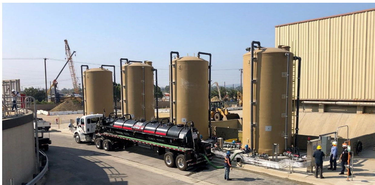
Figure 1. JWPCP’s first slurry receiving station has two offloading stations, each with two storage tanks. Source: LACSD.
