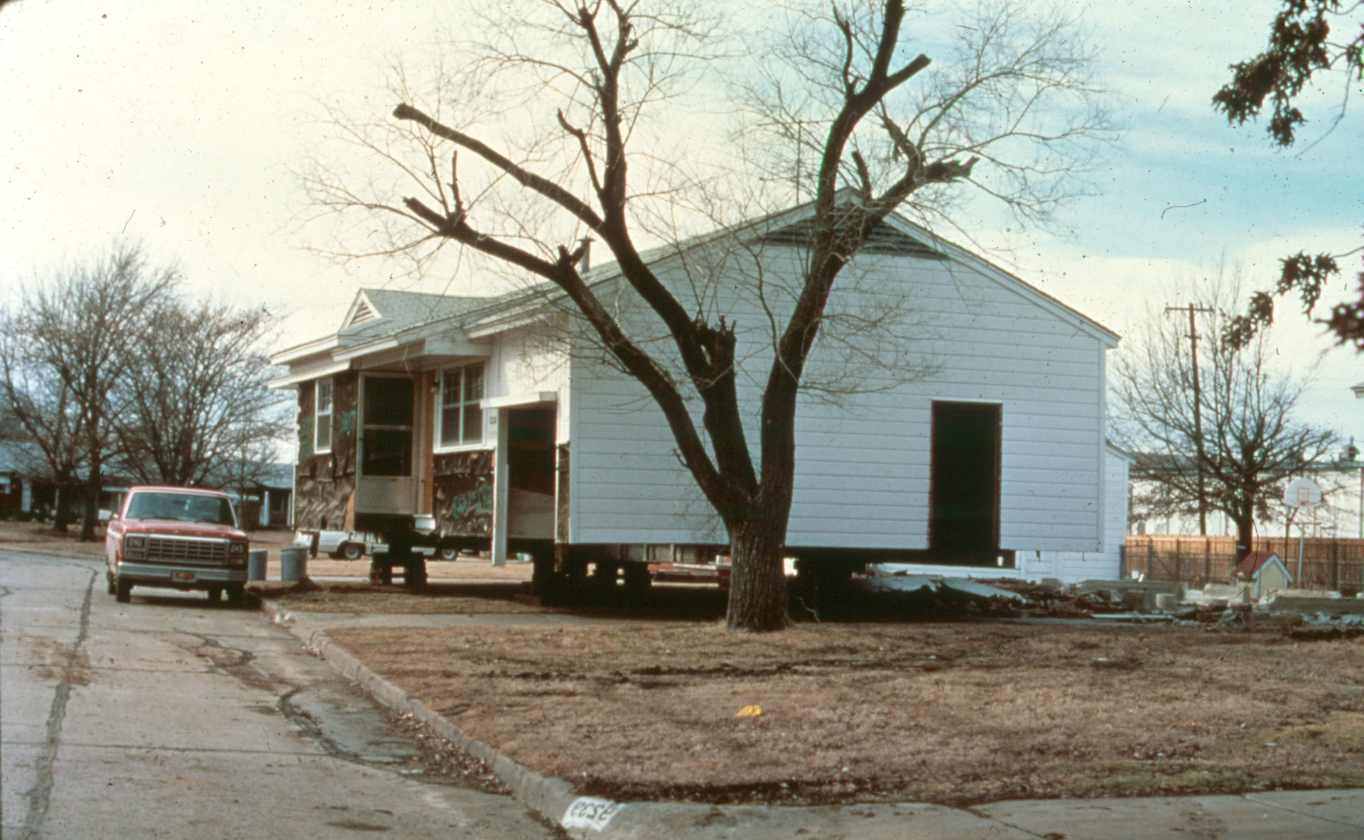
Moving a Flooded House from the Mingo Creek Acquisition Area (1985)
