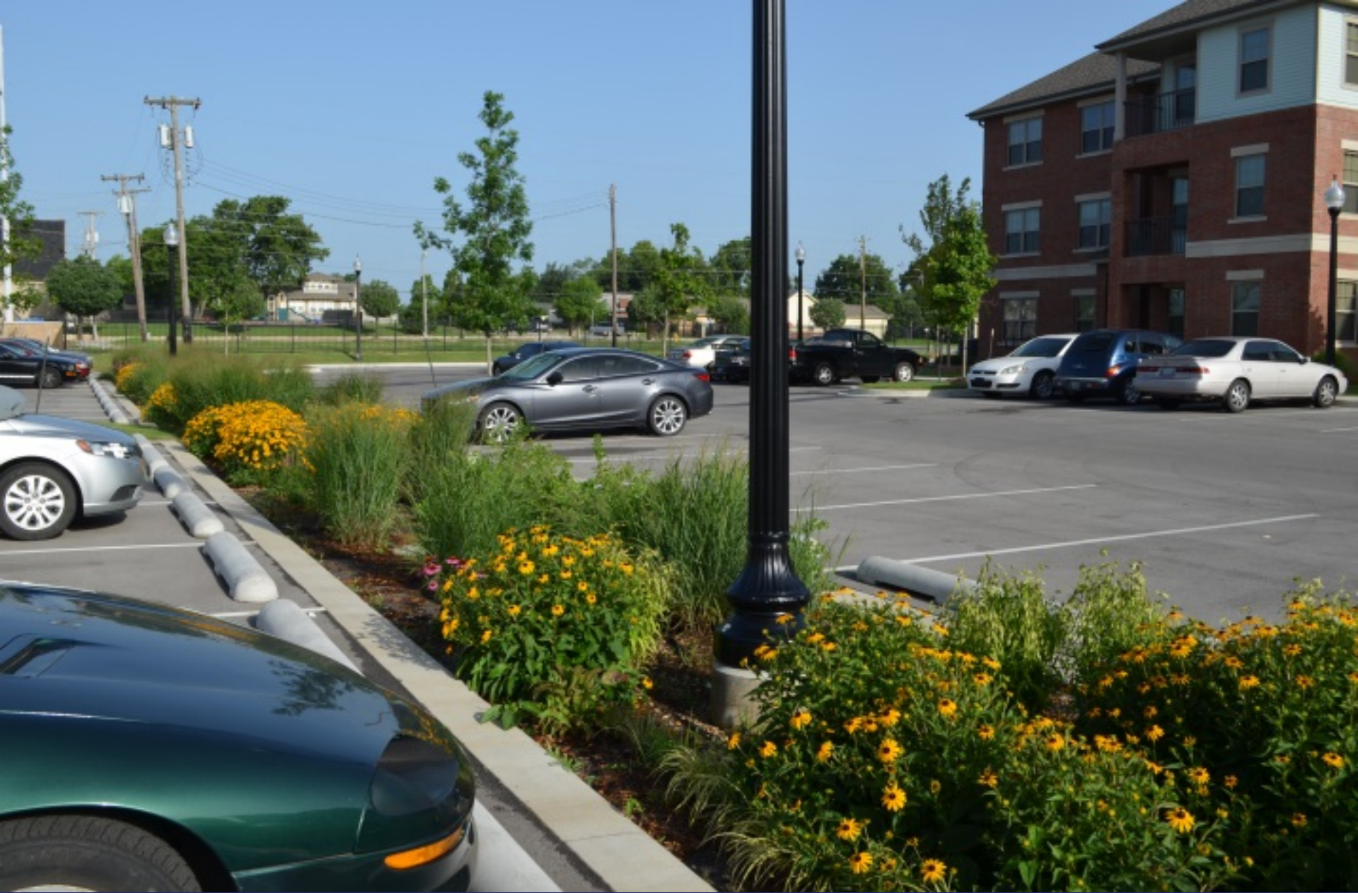
Apartment Parking Lot BioSwale
