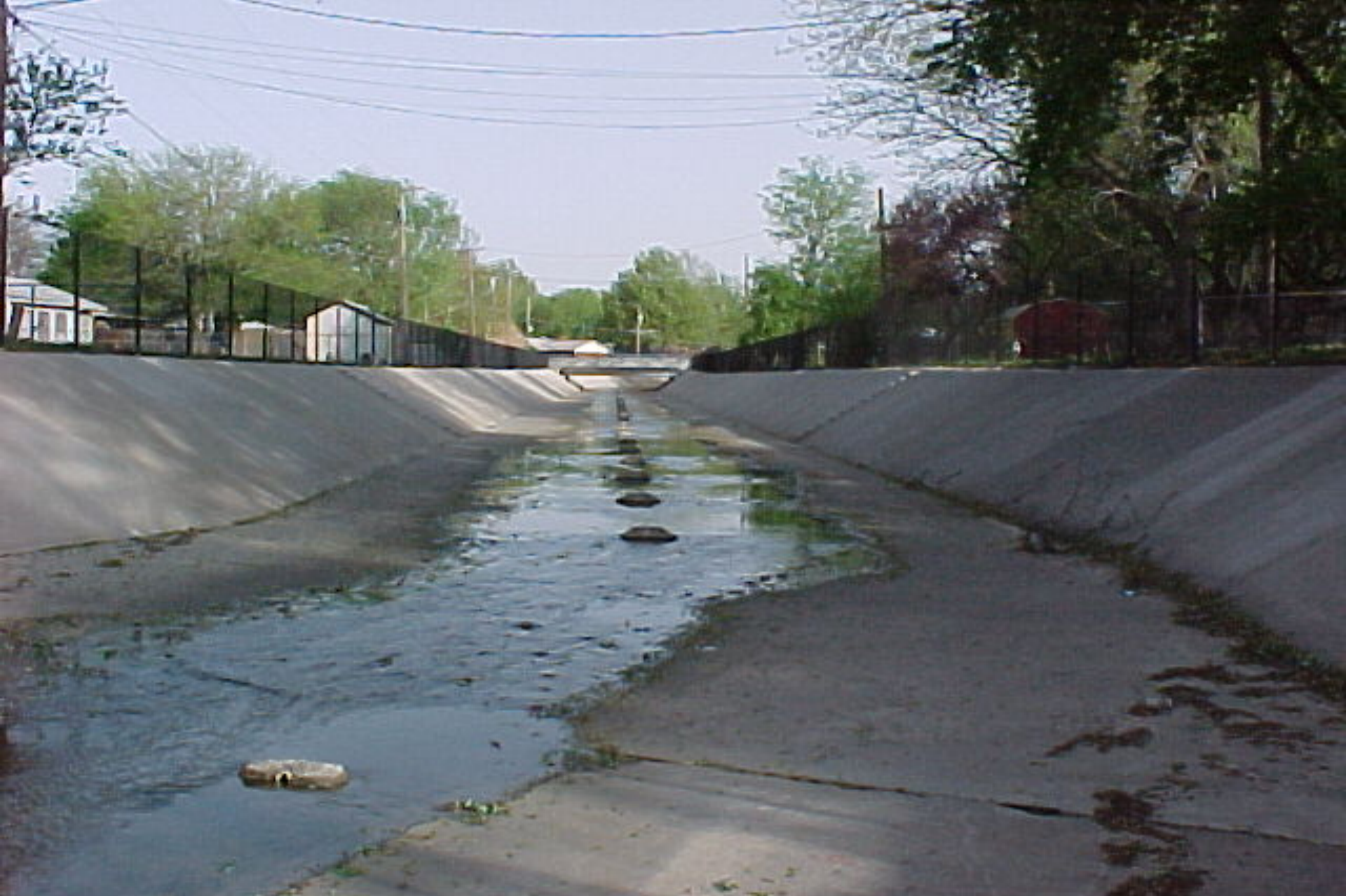
Concrete-Lined Single Purpose Urban Drainage Channel
