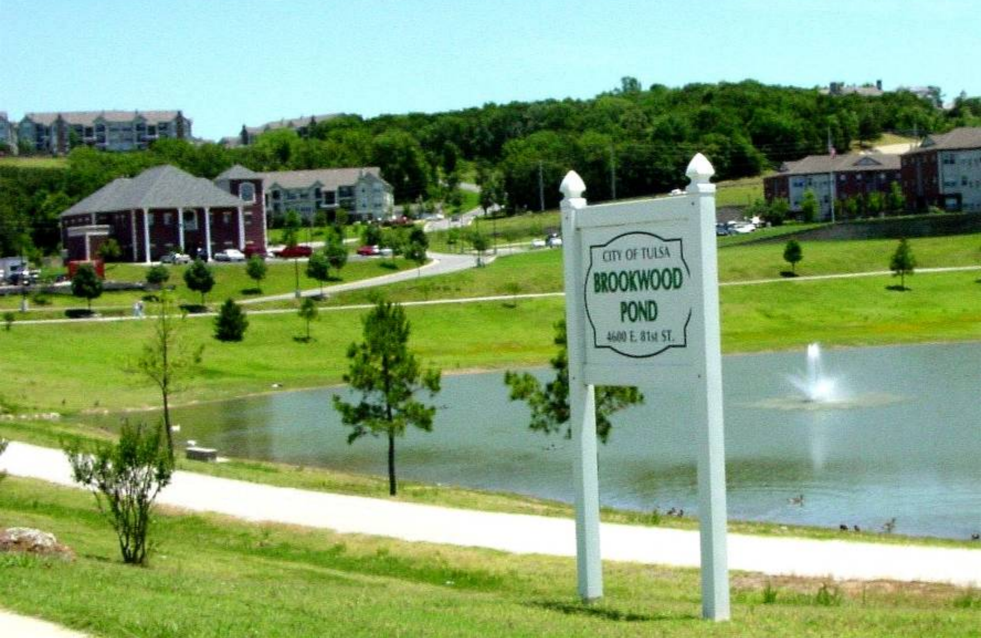
Brookwood Regional Stormwater Detention Facility
