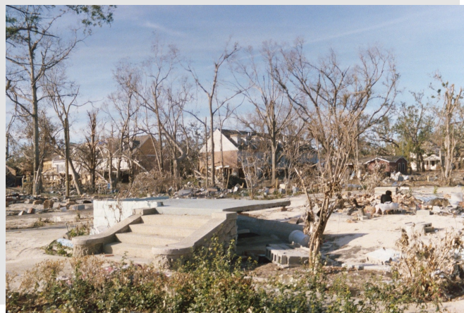
Damaged caused by Hurricane Katrina in Mississippi.
