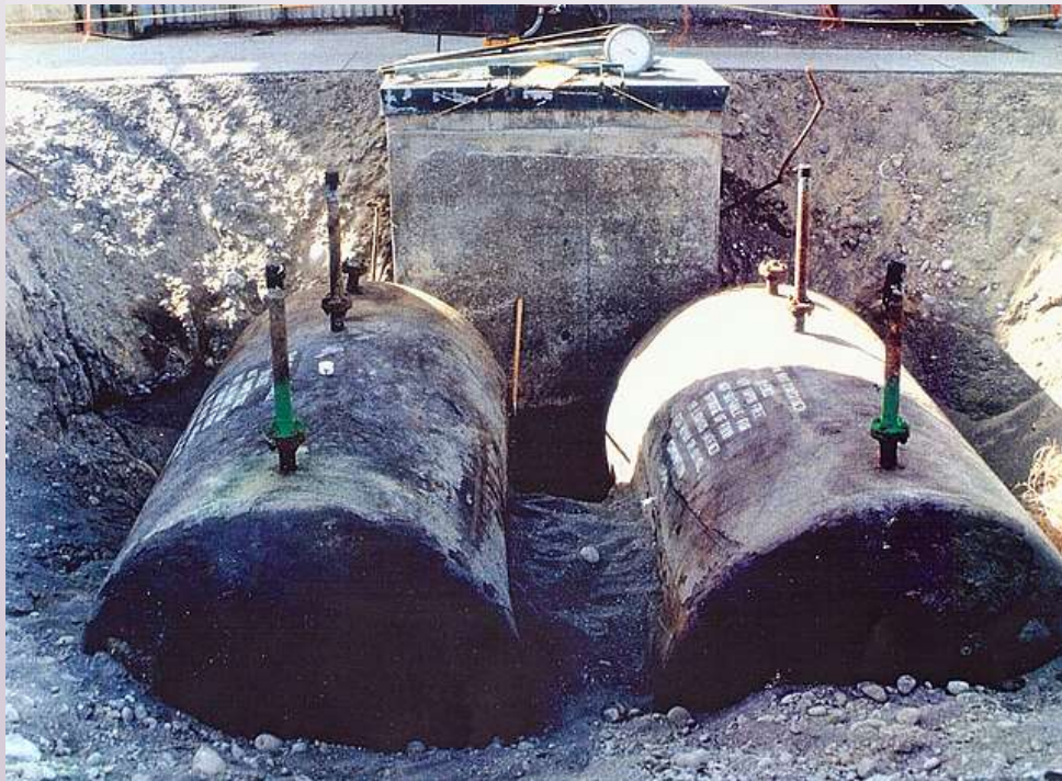
US Dept. of Energy Photo - Underground Storage Tank Removals Typical Excavation
