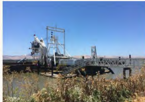
Montezuma Tidal and Seasonal Wetlands Restoration Project
